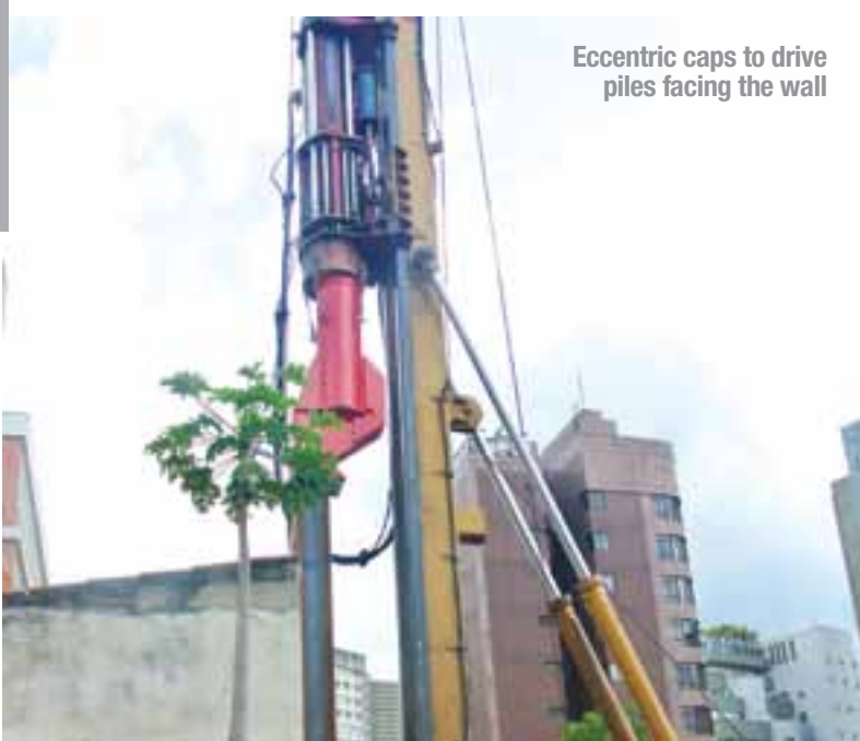
Very compact hydraulic hammer
