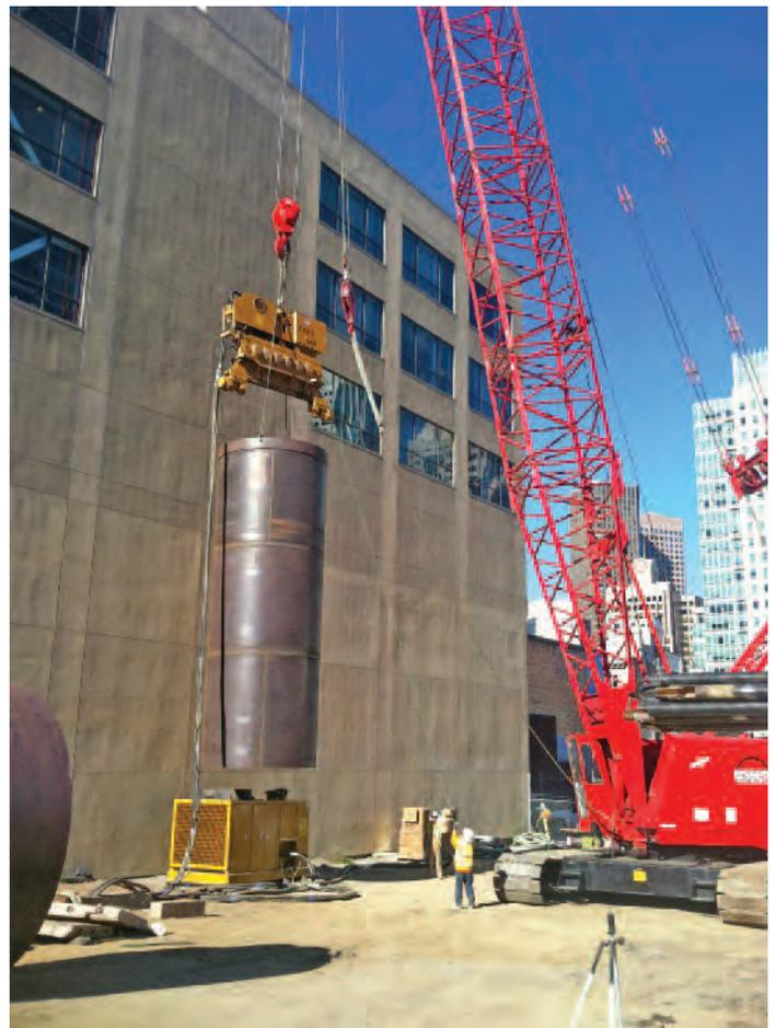
4100 Crane with 200-6 vibratory hammer holding 120” diameter x 30’0” long casing to be installed in Bent 5.
