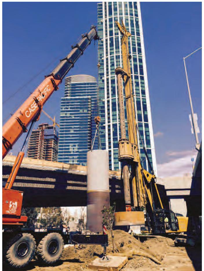
*Bent 20 Permanent casing installation.*
