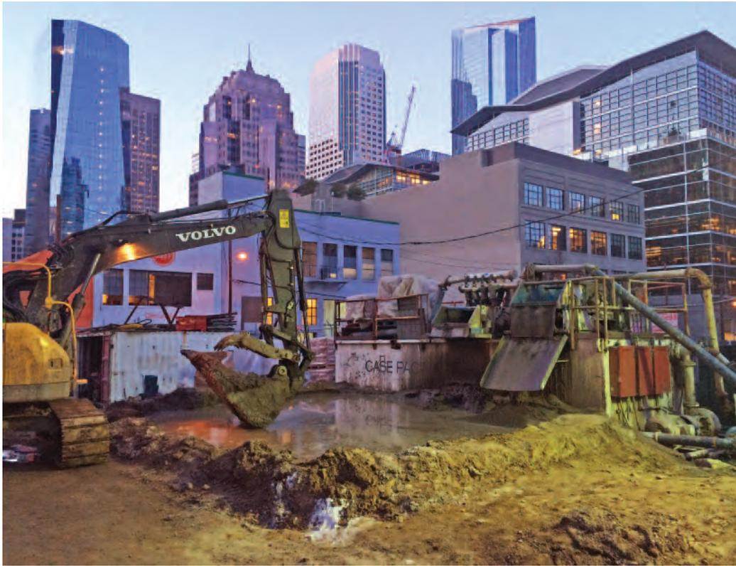
*Mixing and De-sanding Bentonite Slurry System.*
