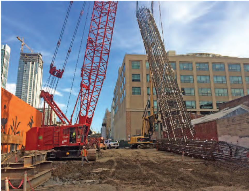
Rebar cages being hoisted into the air with limited clearance from nearby properties.
