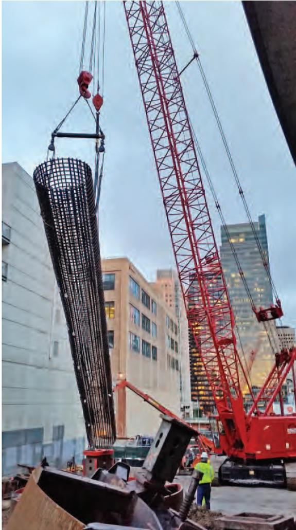
Rebar cages being hoisted into the air within only a few feet clearance from neighboring properties.
